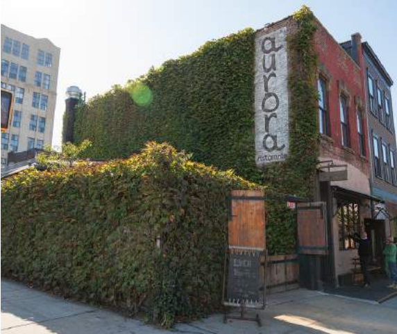
The development sale with the highest price per buildable SF was 70-72 Grand Street/314-326 Wythe Avenue in Williamsburg, which sold for approximately $842 per buildable SF in October.
