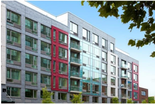
The building at 53 Broadway in Williamsburg was the second largest trade at $59M equal to $722/SF.
